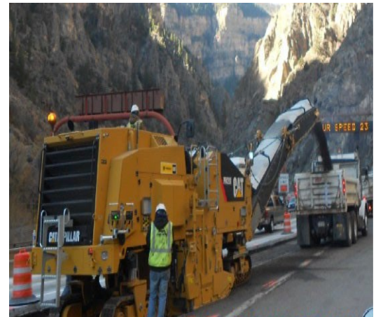
Figure 1. Milling Roadway
